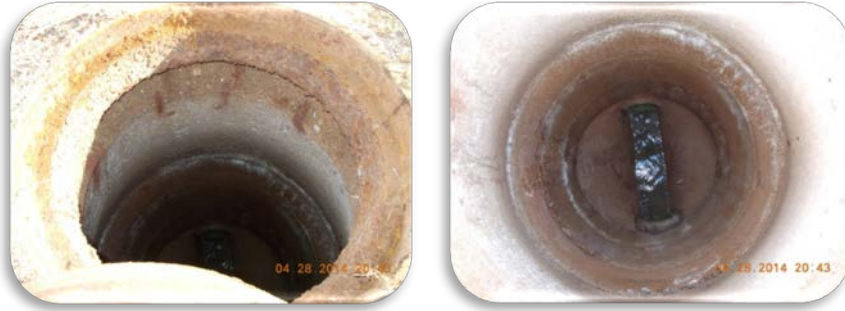
Figure 4-2: Example Manhole Photographs
