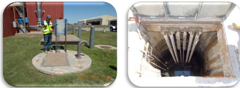
Figure 4-3: Example Lift Station Photographs
