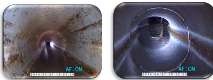
Figure 4-1: Example Pipeline Photographs
